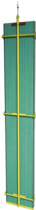
Picture 8. Unloading the panels with the use of a support frame
