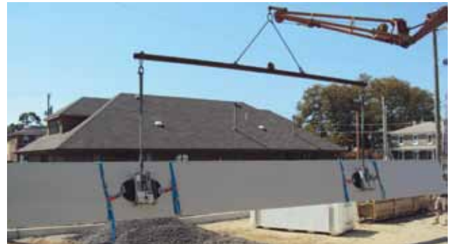
Picture 23. A sandwich panel correctly secured for further assembly.
