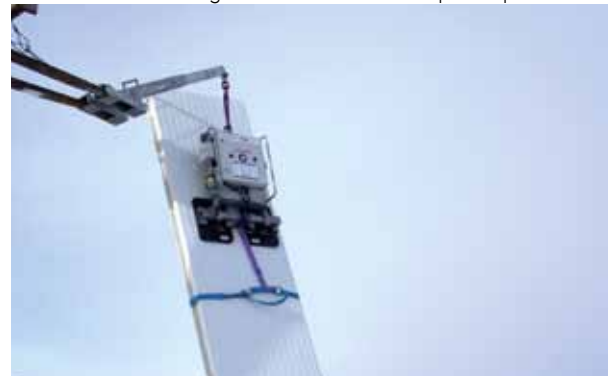
Picture 20. Lifting a correctly secured panel with vacuum cups and belts.
