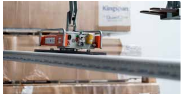
Picture 19. Positioning the elevator on the top/first panel.
