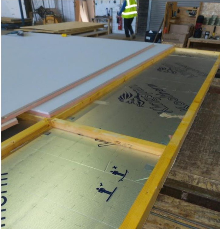
Photograph 4 – View of the insulated plasterboard being fitted to the frame
